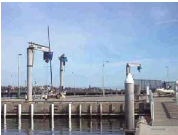
Cranes and pontoon area looking south
